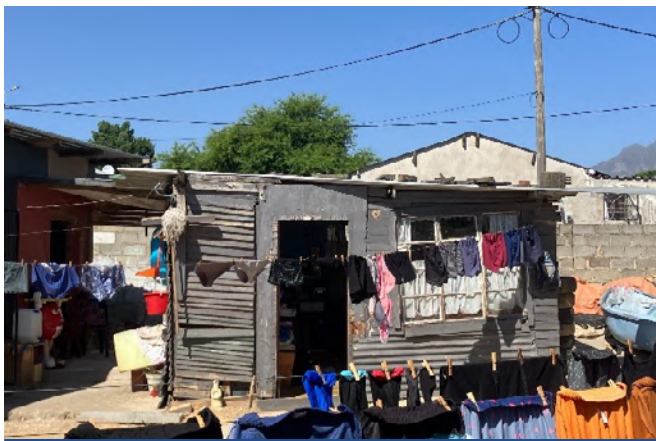
House that does not meet standard
